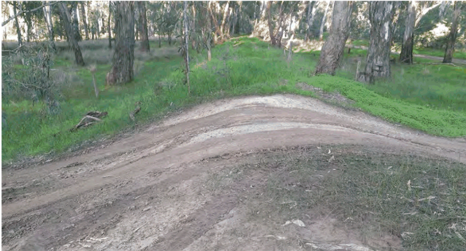
Photo 11: Levee bank construction and traffic - Gemmills Swamp to North Shep (north)
