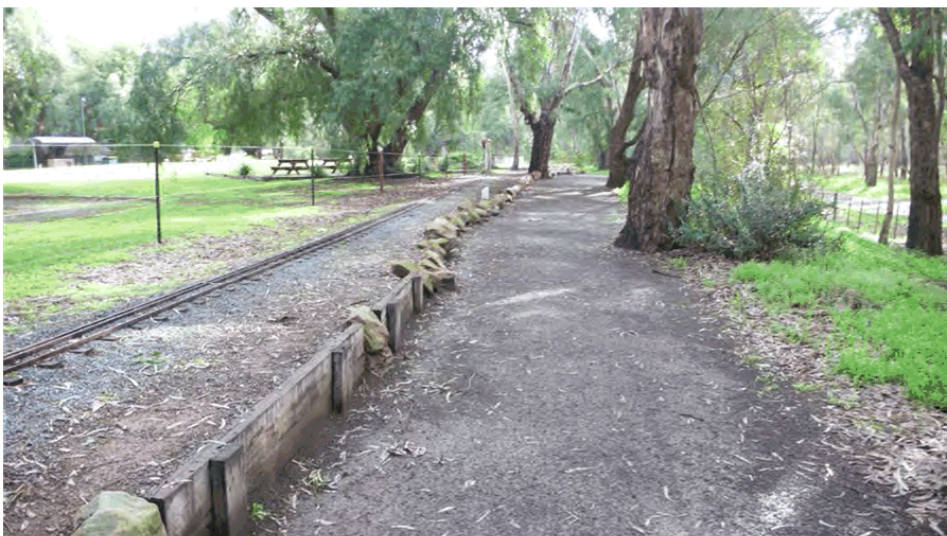
Photo 14: Existing track, retaining wall on Kidstown to Gemmills Swamp path (south)
